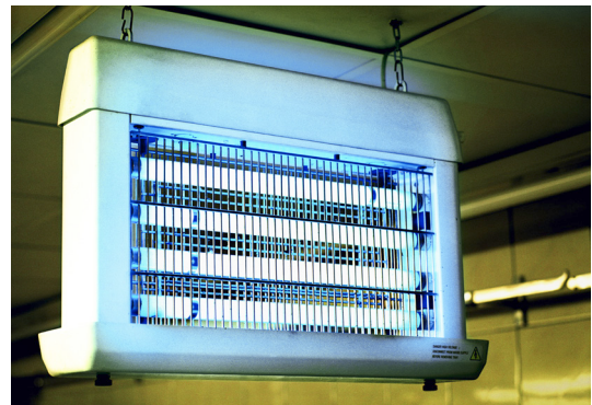
An electric, ceiling-mounted fly killer used for pest control in a kitchen
