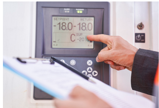
A technician inspecting the temperature of a commercial freezer
