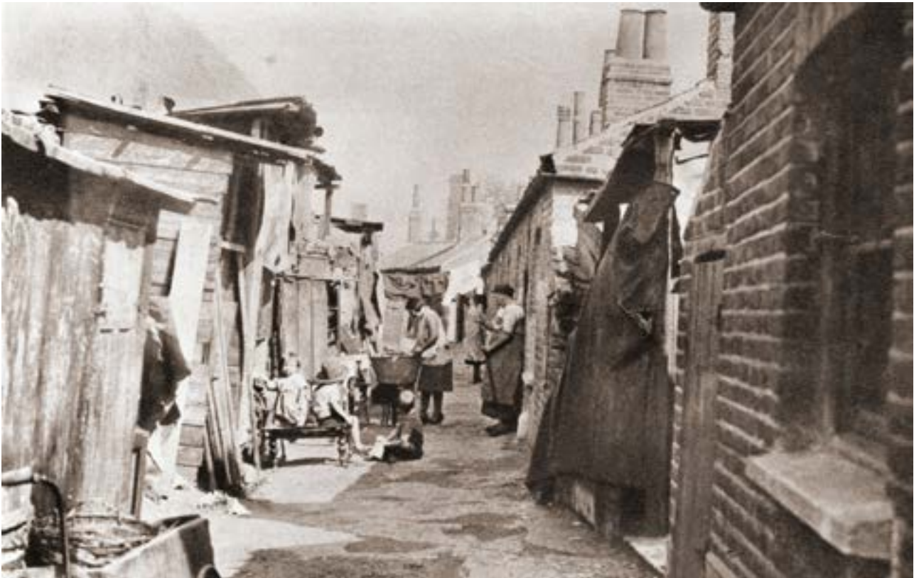
Source E: Slum housing in 1930s Britain.
